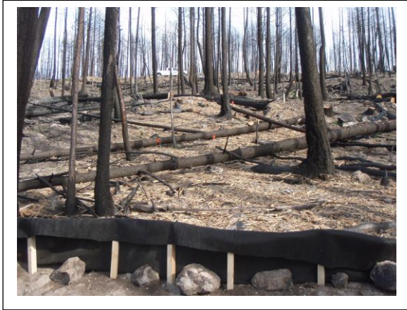
Figure 9: Slope Stabilization. Contour felled log, straw and silt fence to stabilize the slopes to prevent soil erosion and runoff (Source New Mexico State Forestry)
