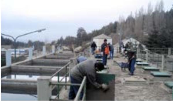
Cleaning filter beds at Bariloche WTP, Argentina after June 2011 eruption of Cordon Caulle, Chile when 30-45 mm ash fell locally. Ash enters sand filter from direct fallout and through intake.
